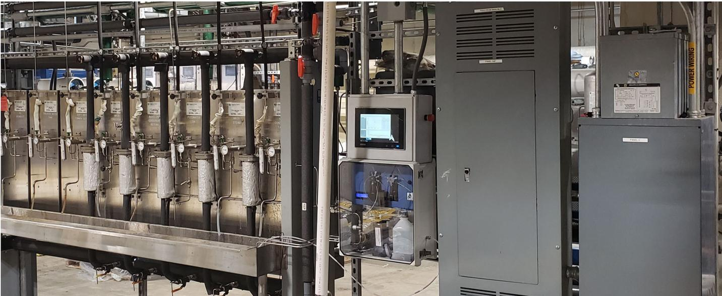
responding table. This system provides automated, on-line, semi-continuous amine monitoring capabilities in your boiler water systems. The measurement provides information on specific amines—not just a total amine level—information that becomes more important when amine mixtures are used.
